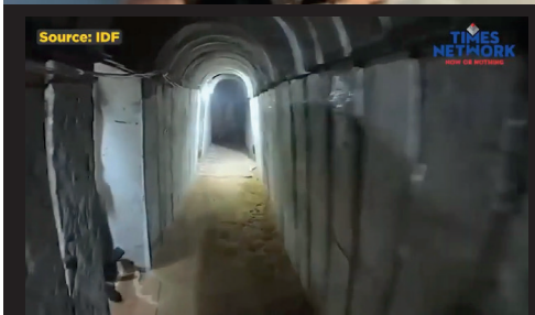
Hundreds of miles of tunnels found
